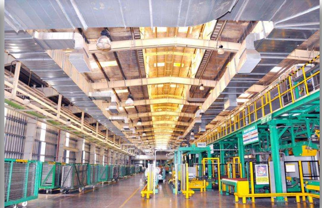
***Maximum utilization of Day light as a substitution of Electrical light in day time by installing transparent acrylic sheets.***
