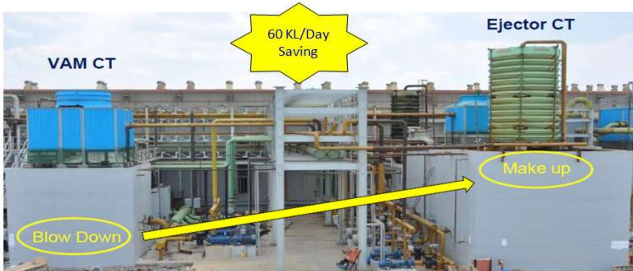
VAM CT Blow Down used as Ejector CT Make up to reduce Fresh Water Consp.
